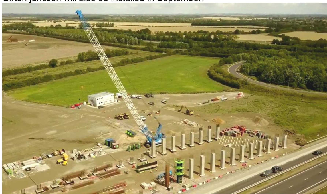
Bridge columns under construction next to A428.
